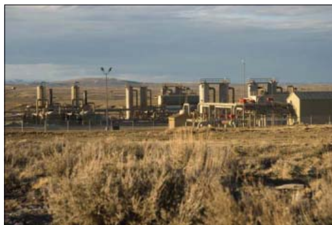
Enterprise Products Partners LP's silica gel gas plant sits next to the company's newly opened Pioneer natural gas processing plant in Sublette County, Wyo. Pioneer began operations in February 2008 and will eventually process about 525 MMcf/d from the Enterprise-operated Jonah gas gathering system and extracting about 25,000 b/d NGL. The plant is designed to process up to 750 MMcf/d and extract as much as 30,000 b/d. Enterprise will continue to operate the silica gel gas plant as backup, it said, as was needed in late March when a gas leak and fire closed the Pioneer plant for several days. Photo from Enterprise.
