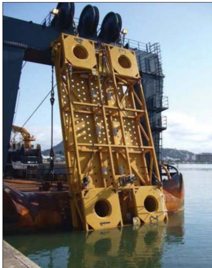
The spacer template for an artificial lift manifold (ALM1), built by FMC CBV Subsea, is secured on the A-frame of an anchor-handling vessel, before installation (Fig.4; photo from Shell).
